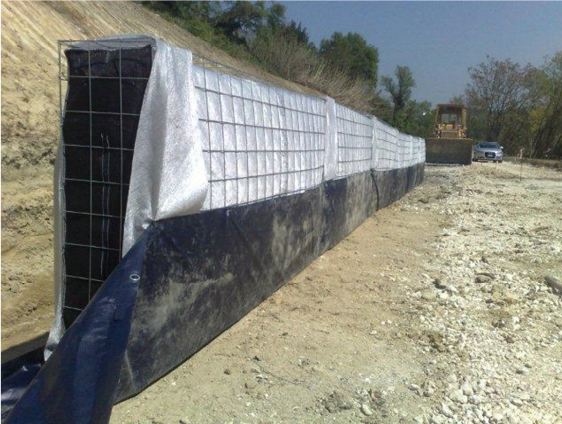
Fig.4-DRENTER modules mounted along the trench of the first drain
