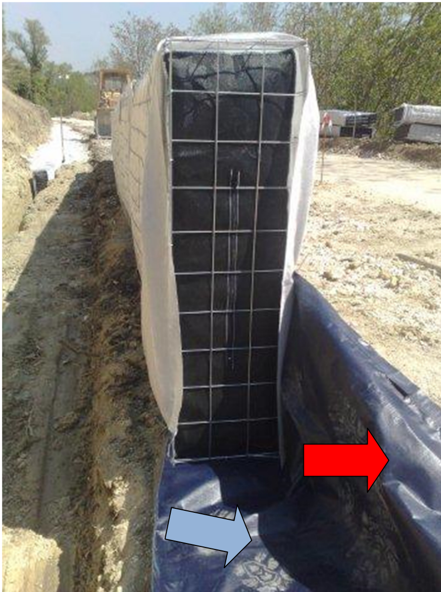
Figure 3-Laying the liner and draining panels along the trench for the drainage, note the liner positioned at L
