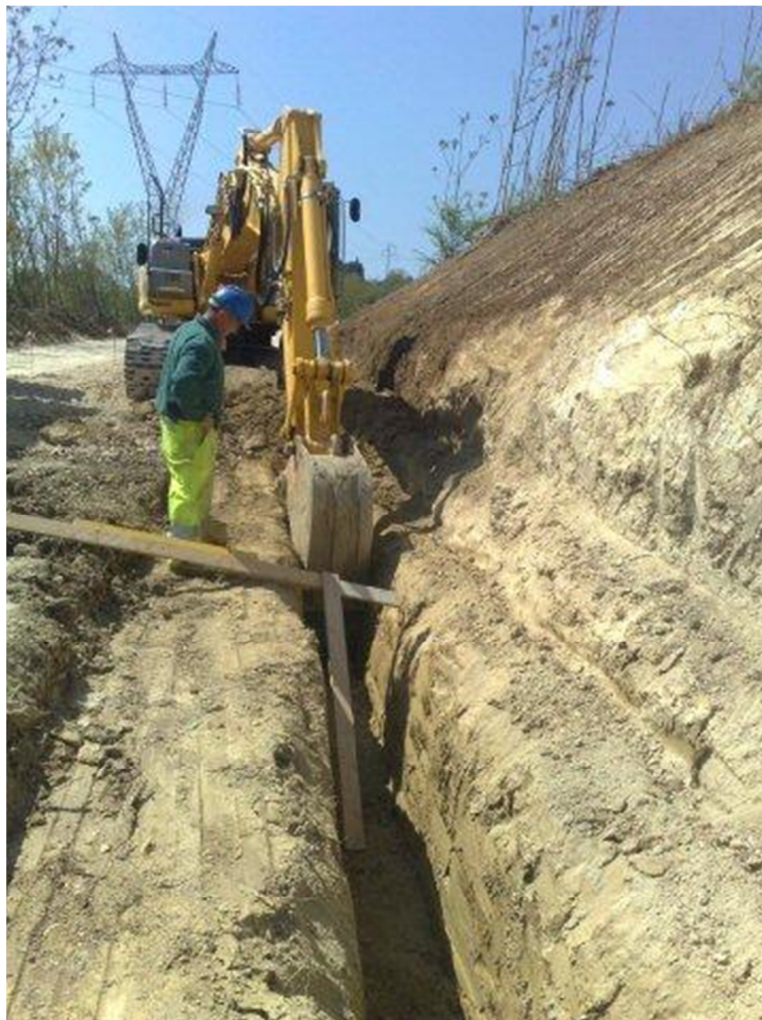
Figure 2 - excavation carried out with a mechanical excavator for the installation of the DRENTER system
