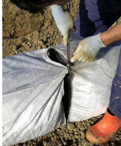
After the binding on the four vertices, the joint is covered by a non-woven geotextile band to avoid soil infiltration in the joints.
