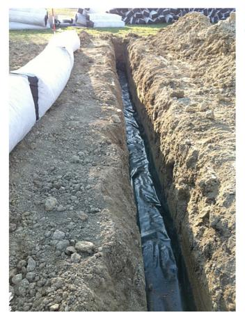
To guarantee the hydraulic continuity of the drain, an impermeable sheath is applied to the bottom of the excavation, which in this case has been fixed to the walls with nails (Fig. 2).
