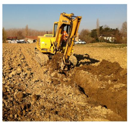
The choice of the 0.40 m bucket is to ensure the maintenance of the ideal section of the modules, which is remembered having dimensions of 0.3x0.5 m, once lowered into the trench (Fig.1).
