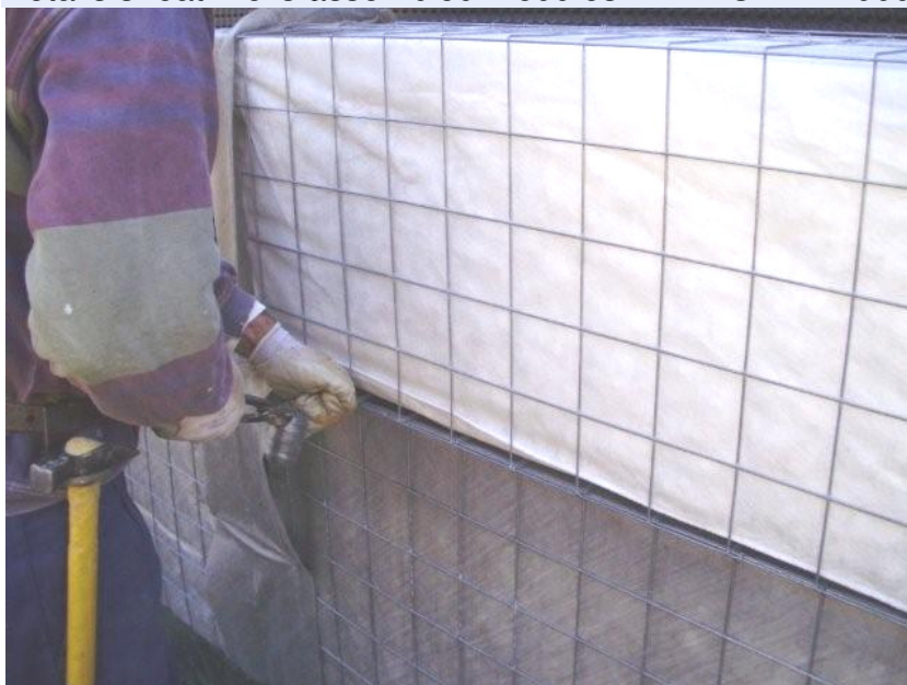
Fixing core modules DRENTER 500 with modules DRENTER 1000
