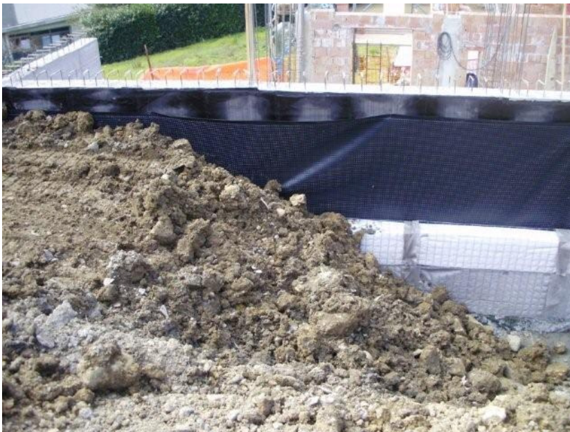
Phases of the modules DRENTER backfilling with soil excavated natural
