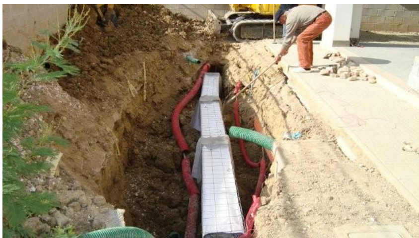
FIG. 4 Draining on installation
