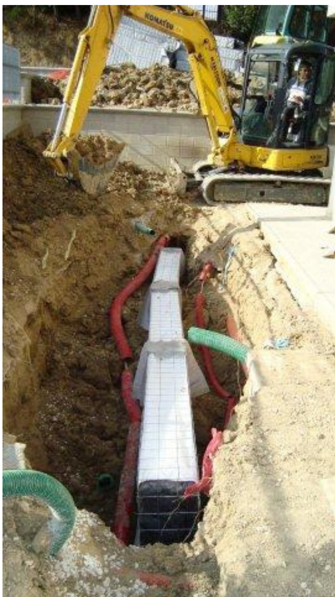
Filling of the trench with excavated soil
