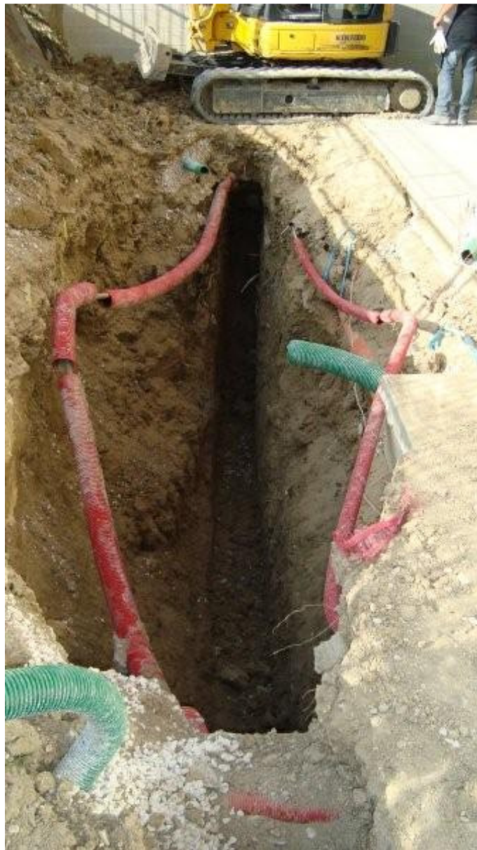
FIG 1 Narrow excavation
