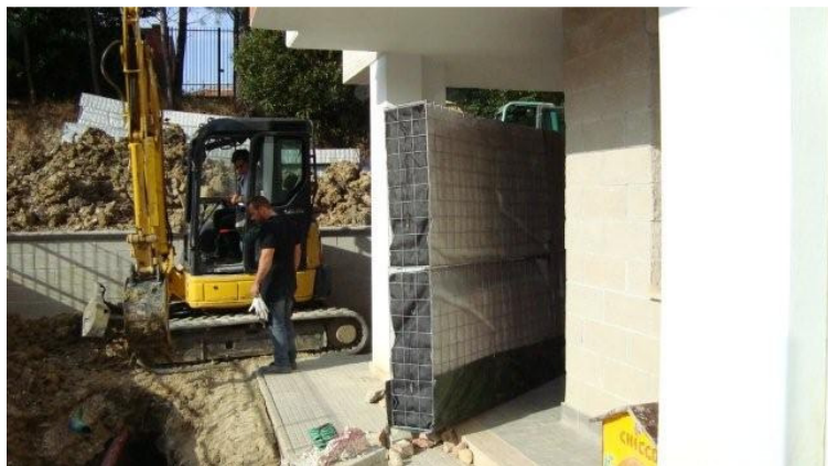
FIG. 3 Draining waterproofed strip ready to be placed inside the trench.
