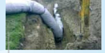
once all the products have been put in place, the trench is filled in with the spoil, which must cover the module with a layer of soil about 30-50 cm deep.
