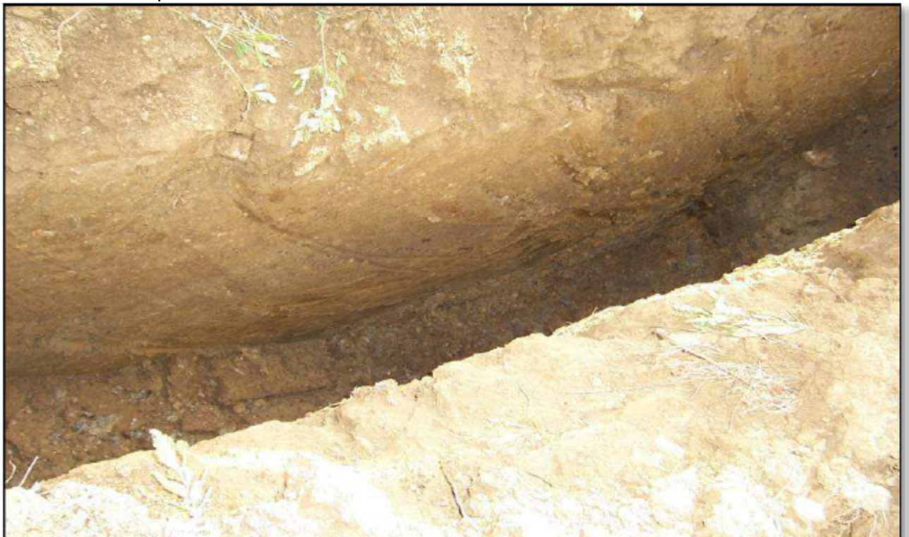
Figure 3 - Excavation with a mechanical excavator for the installation of the IDROSAC 500 system at the Montalcino estate (SI).
