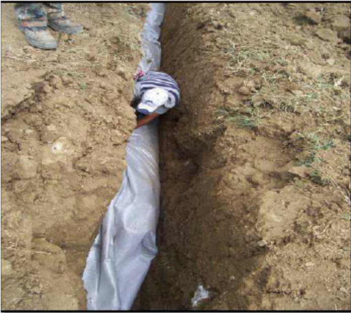
Figure 6 – Lining operation draining bags with the TNT carried out manually inside the trench
