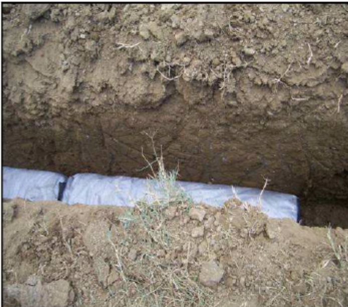
Figure 4 - Pieces of geotextile of the type non-woven fabric (TNT) used for cover IDROSAC 500 draining bags at the estate in Montalcino
