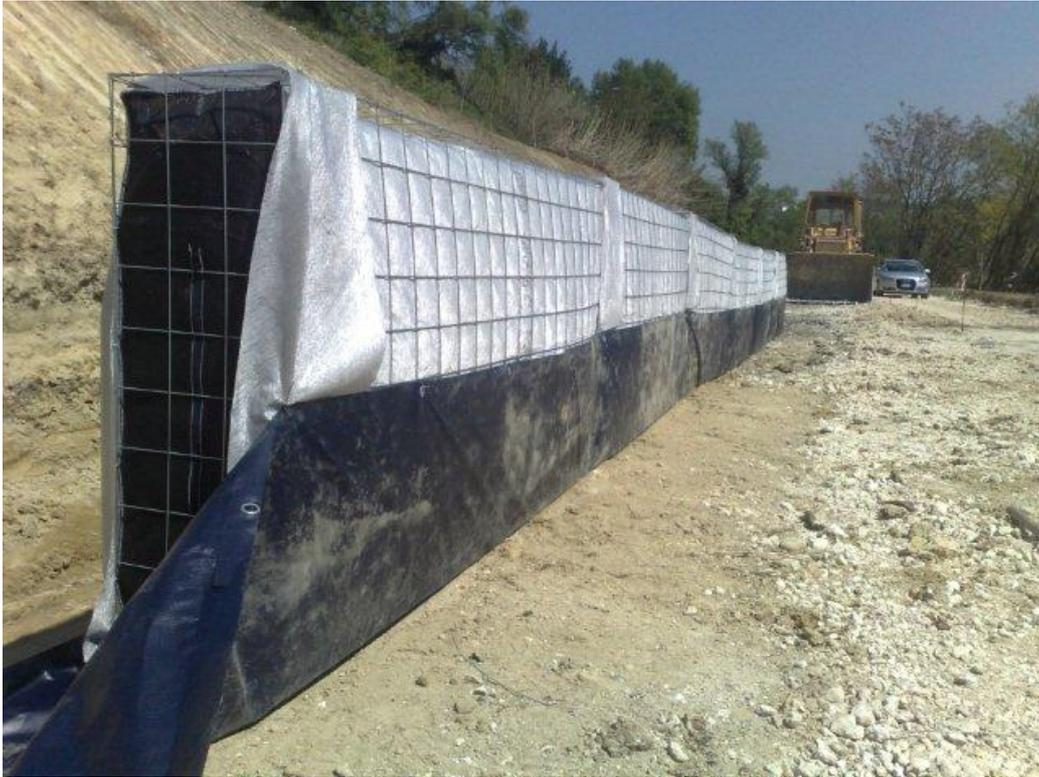
Figure.4-Logement du system DRENOTER.
